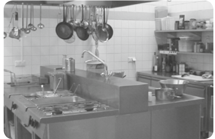
Filter monitoring in kitchens
